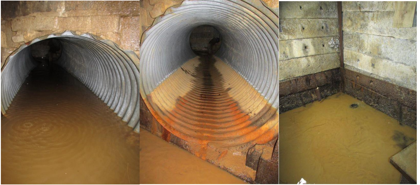
View of the entrance to the lower chamber before and after clearing the drain
